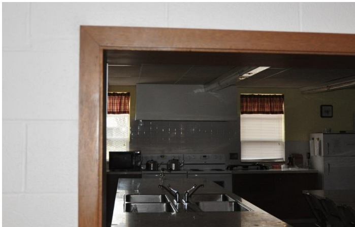
1 Remove casing from jamb if present. Shutter needs to be mounted on a flat surface.
